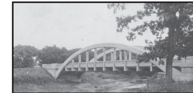
Marsh Rainbow Arch Bridge in Boone County on 210th St.
