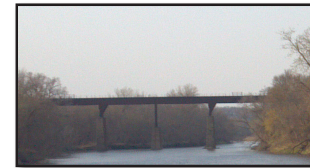
High Bridge in Greene County
